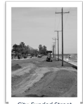
City-Funded Street Development
