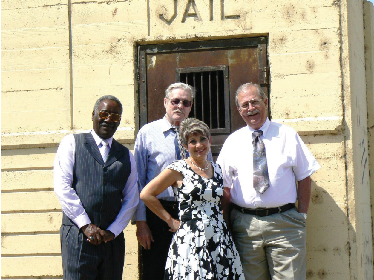
This two-cell jail was built in Buttonwillow, CA in 1940. It remained in service till the late 1960's.
