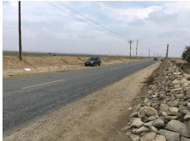
Same section of Panama Road – December 2016
