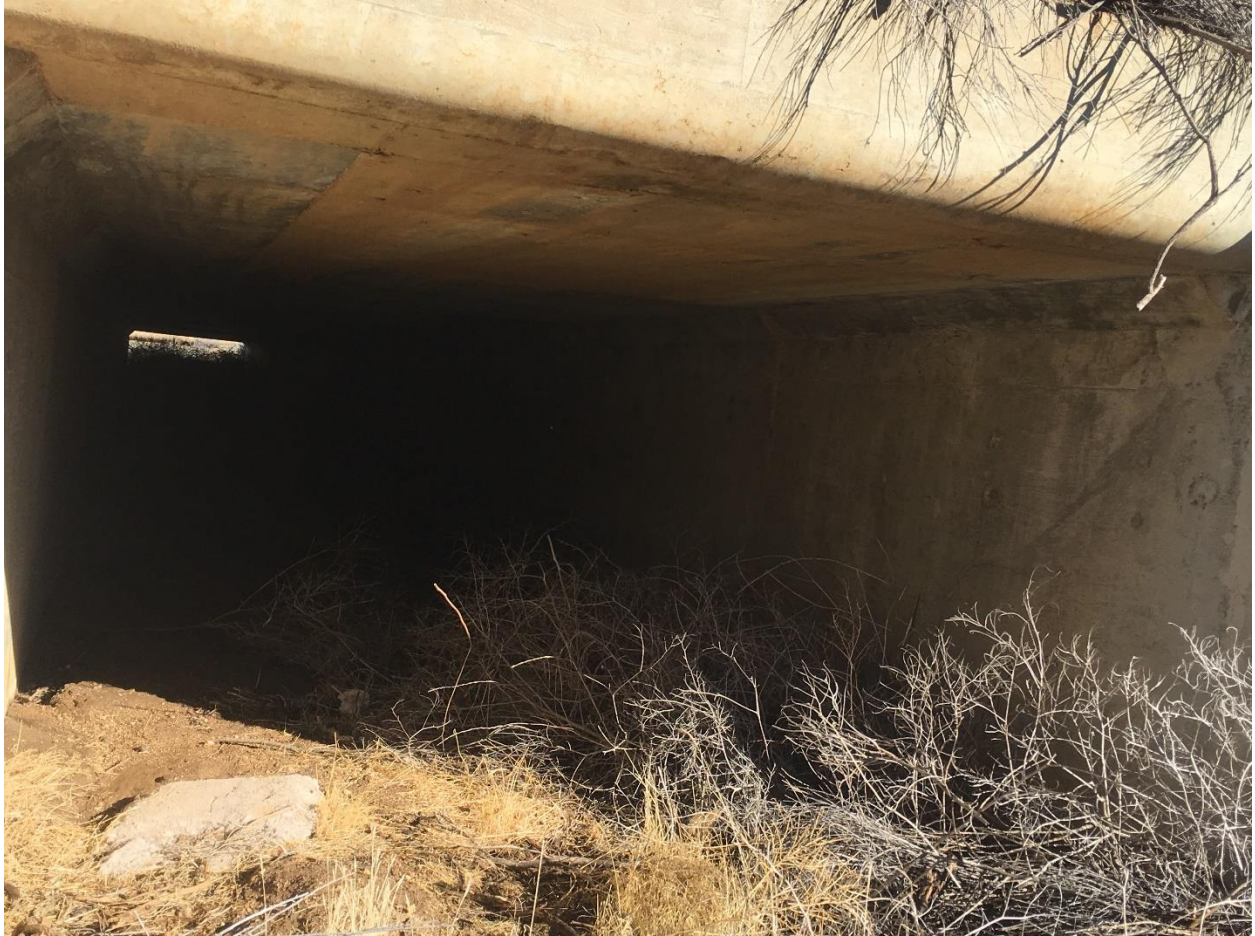
Mountain Meadows Culvert Photo taken by Committee
