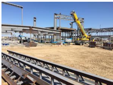
CTEC under construction
