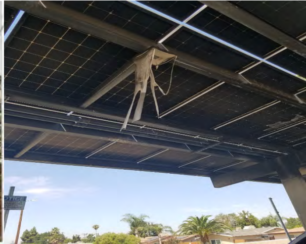
Photo by Grand Jury/ Fire damaged solar & lighting
