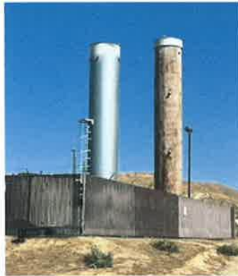
Two stacks at Bena flare off methane gas from sealed landfill cells. (Grand Jury Photo)
