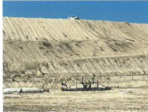
At left, an active landfill cell at Bena. At right, a new cell that will soon have an impermeable lining in preparation for receiving waste. (Grand Jury Photos)
